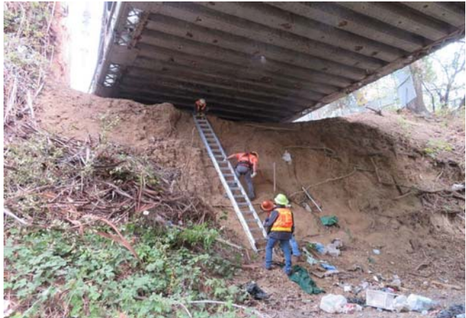
Photo 3 - Inspection crew setting ladder via north side
