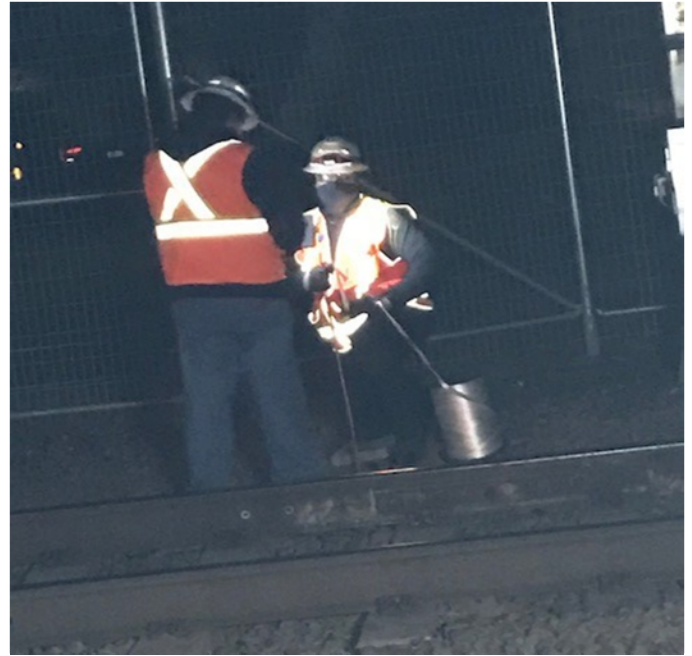
Photo 2 - Workers putting in new signal wires for the train detection in the rail
