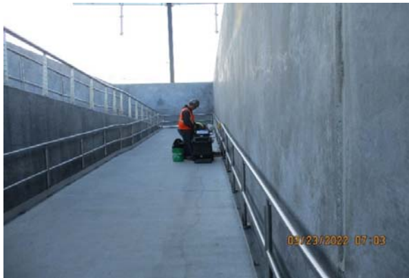
Photo 3 - South Ramp fixing plate kickers
