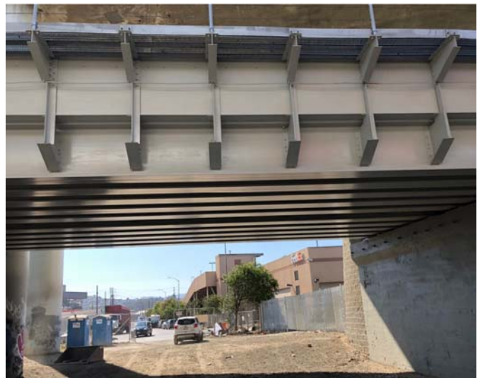
Photo 4 - New Napoleon Bridge
