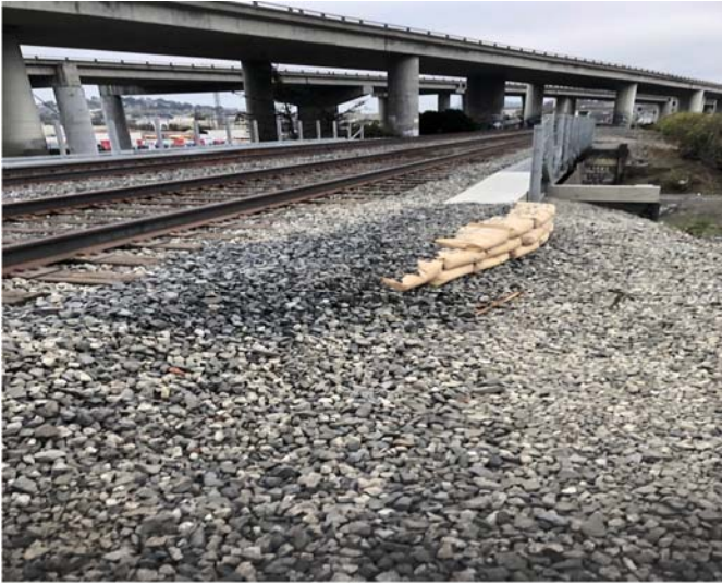
Photo 1 - Marin Street New Walkways
