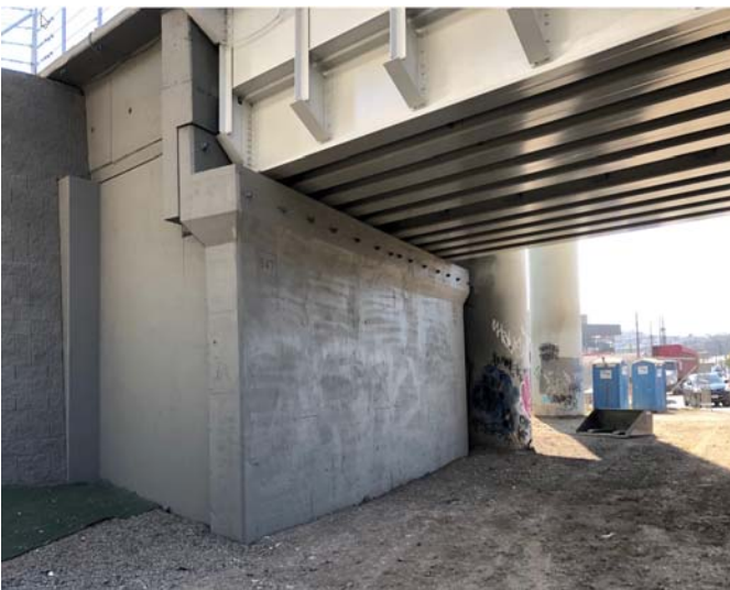
Photo 3 - Napoleon South Abutment
