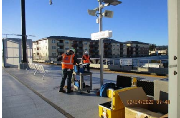
Photo 2 - OCS Grounding Testing.
