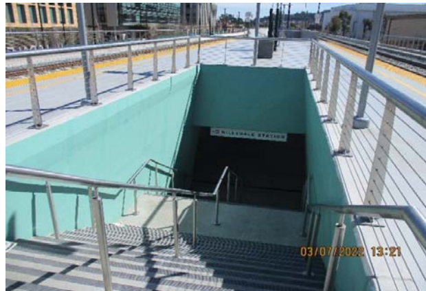
Photo 4 - Stairs Paint Touchup at Hillsdale Station
