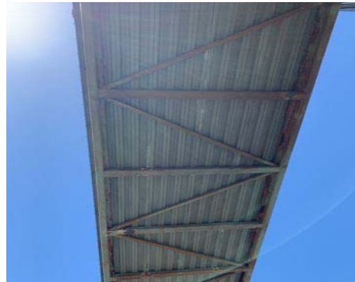
Photo 2 - Pedestrian bridge (underside)
