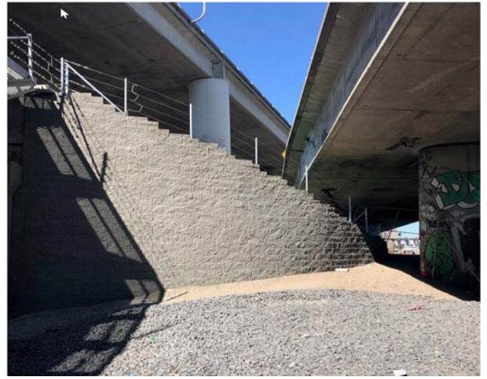
Photo 2 - Napoleon Northeast Retaining Wall
