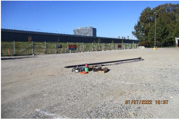
Photo 1 - 25th N Yard Lighting Pole
