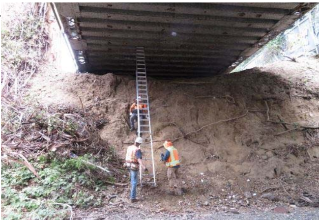
Photo 4 - Inspection crew via north side abutment
