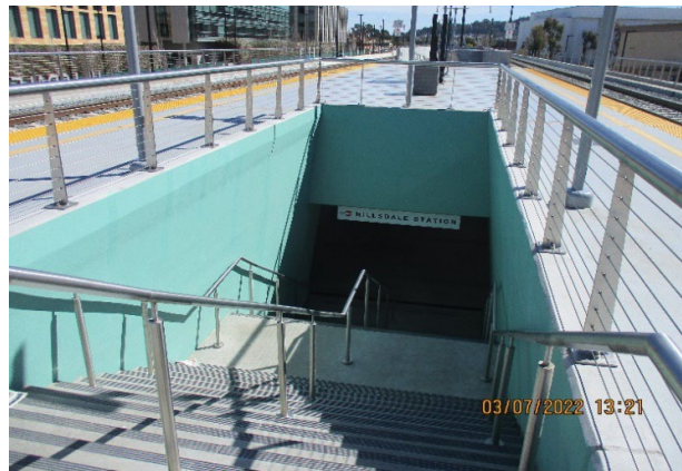
Photo 4 - Stairs Paint Touchup at Hillsdale Station
