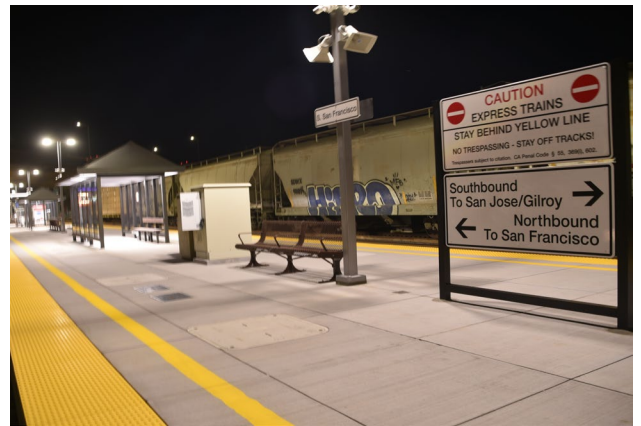
Photo 4 - New platform signage
