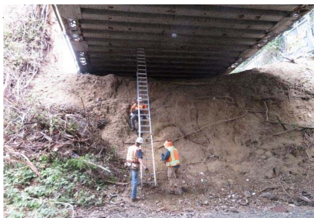
Photo 4 - Inspection crew via north side abutment
