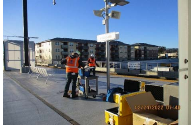
Photo 2 - OCS Grounding Testing.
