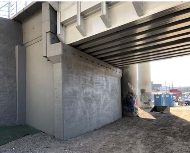
Photo 3 - Napoleon South Abutment
