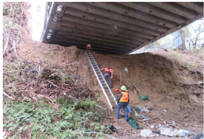
Photo 3 - Inspection crew setting ladder via north side
