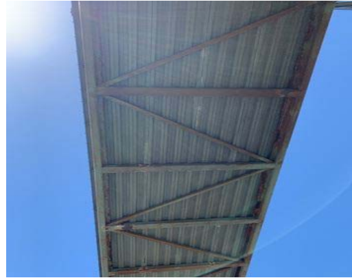
Photo 2 - Pedestrian bridge (underside)
