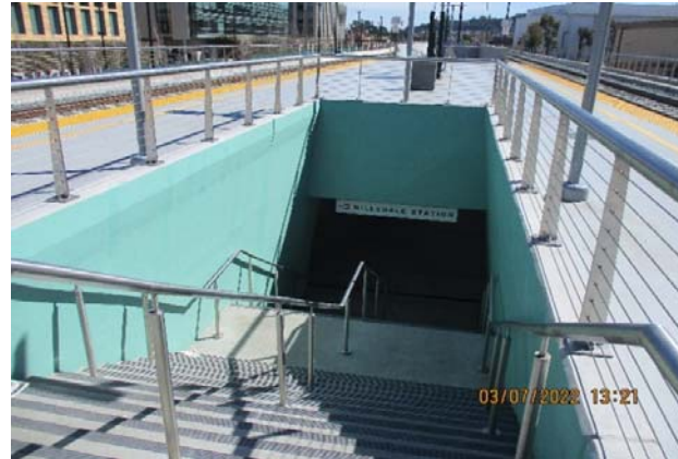
Photo 4 - Stairs Paint Touchup at Hillsdale Station
