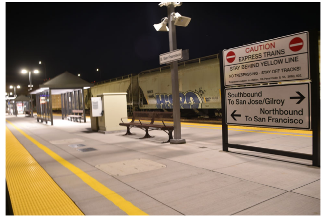
Photo 4 - New platform signage
