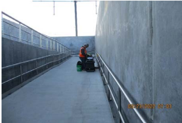
Photo 3 - South Ramp fixing plate kickers
