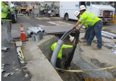
Routing from Splice box to termination point
