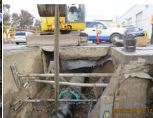
Water main tie in East Grand Ave.
