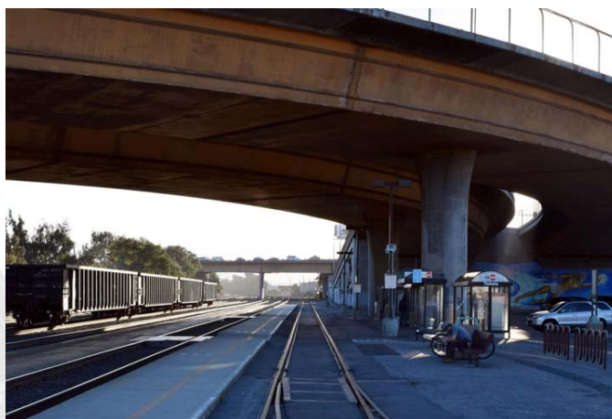
Existing Platform – South San Francisco Station Boarding
