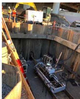
Shoring and Main installation - West Plaza
