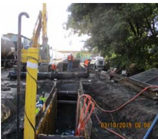
18 inch water main East side UPRR track
