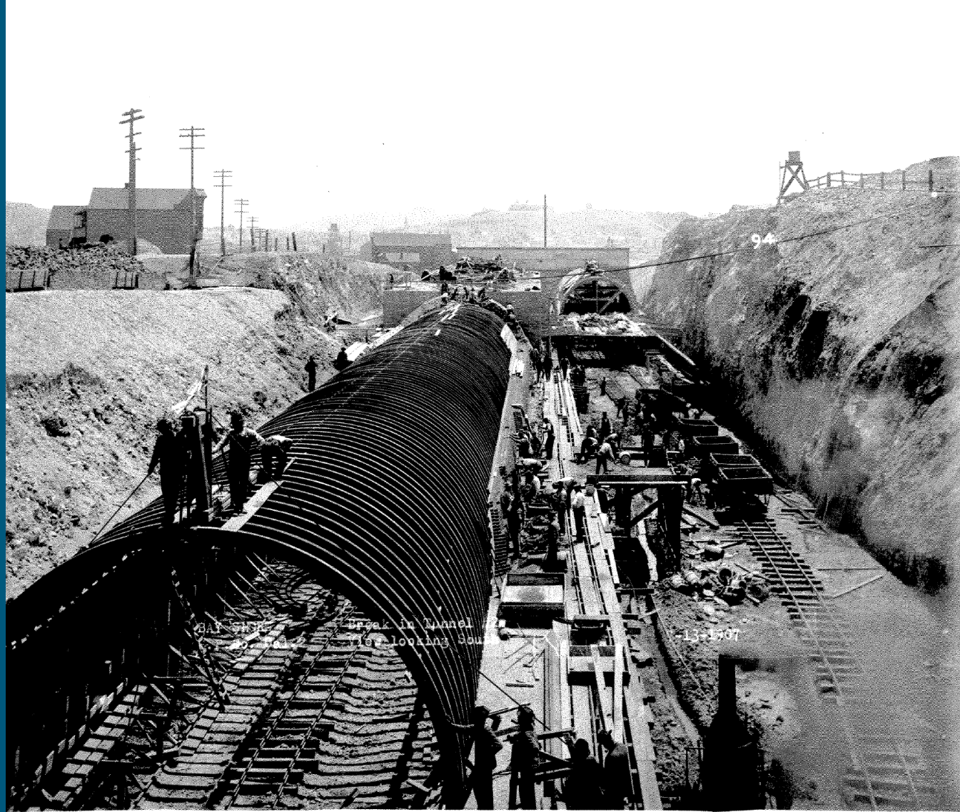
Bayshore Tunnels under construction, 1907
