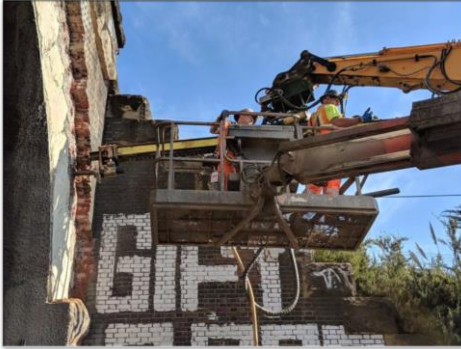
Installation of Canopy Tubes for Steel Set Reinforcement
