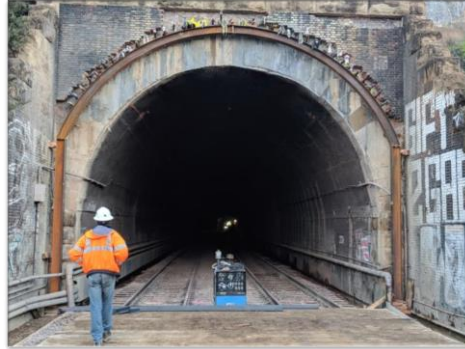
Steel Set Installed
