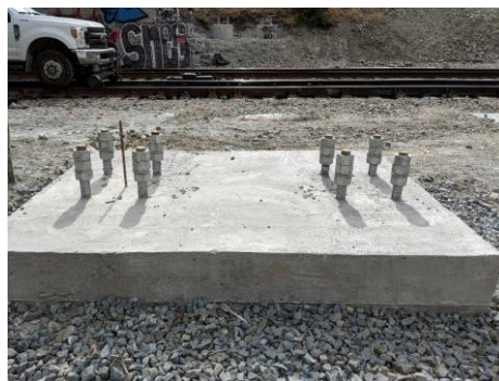
Micropiles and Cap Foundation
