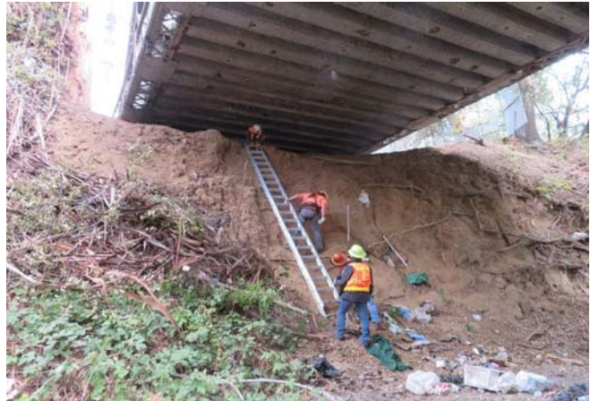
Photo 3 - Inspection crew setting ladder via north side
