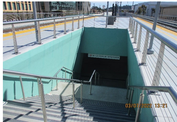
Photo 4 - Stairs Paint Touchup at Hillsdale Station
