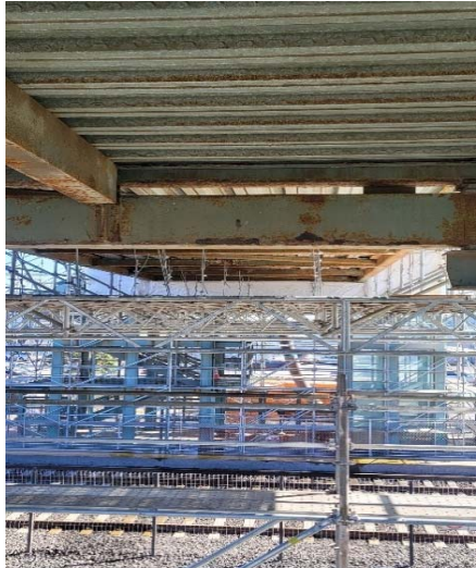
Photo 4 - Bottom view between pedestrian bridge and scaffolding containment system
