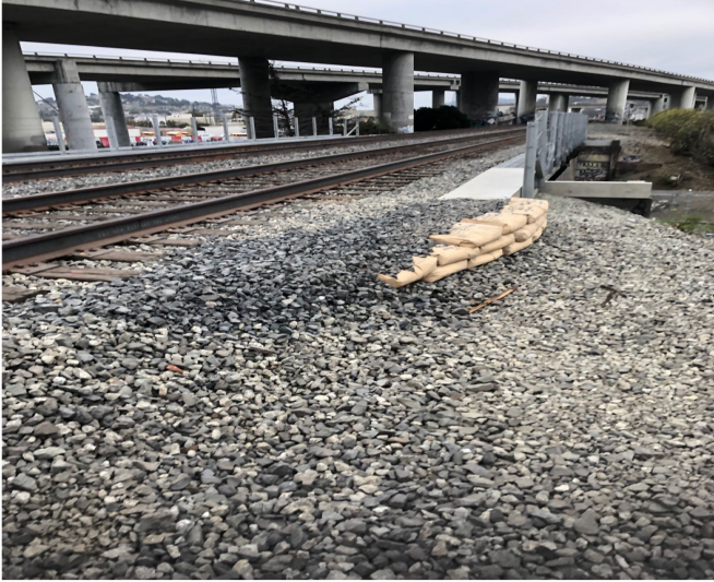
Photo 1 - Marin Street New Walkways
