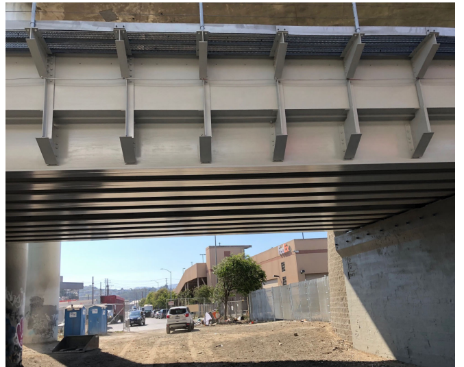
Photo 4 - New Napoleon Bridge
