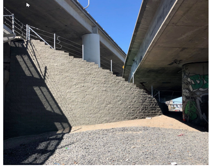
Photo 2 - Napoleon Northeast Retaining Wall
