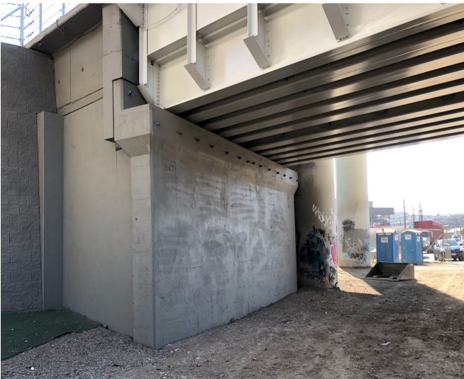
Photo 3 - Napoleon South Abutment
