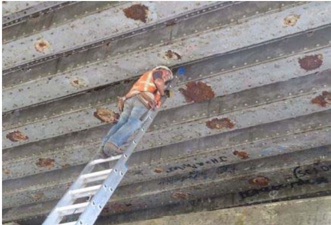
Photo 1 - Inspection crews via underside of bridge via south side
