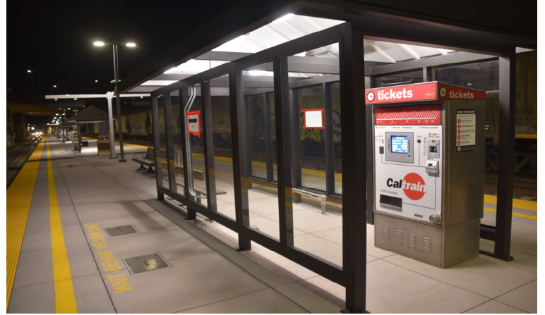
Photo 2 - Shelter with ticket machine
