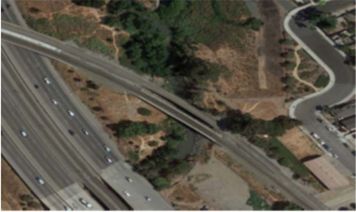
Photo 1 - Aerial View Caltrain MT1 & MT2 Bridges near SR 87 in San Jose
