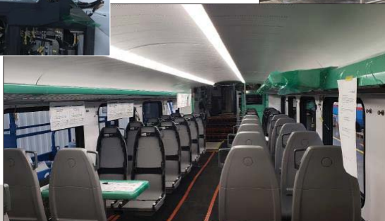
Lower level luggage racks, ceiling, seat frames installation
