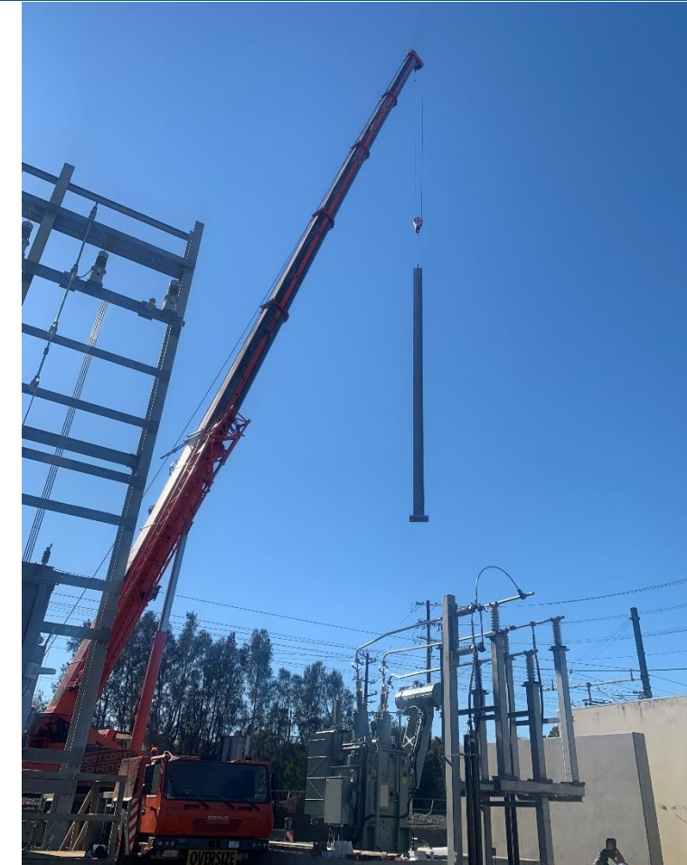
Gantry Installation at Paralleling Station 3
