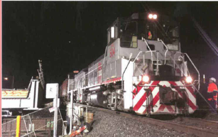
Schedule Changes Will Allow for Vital Caltrain Construction Work
