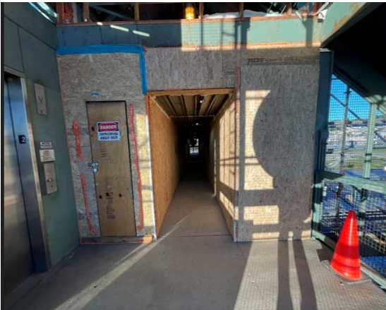
Photo 1 - Pedestrian Bridge Tunnel Containment
