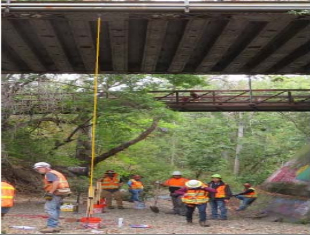
Photo 1 - Pendulum Hung from Bridge
