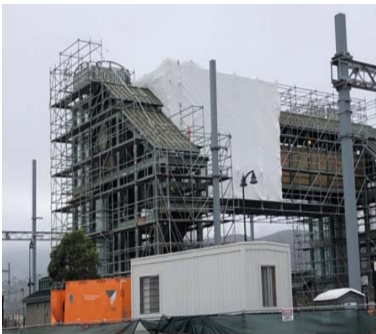
Photo 3 - South Side View of Scaffolding Containment System
