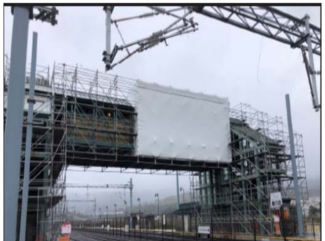
Photo 4 - North Side View Scaffolding Containment System
