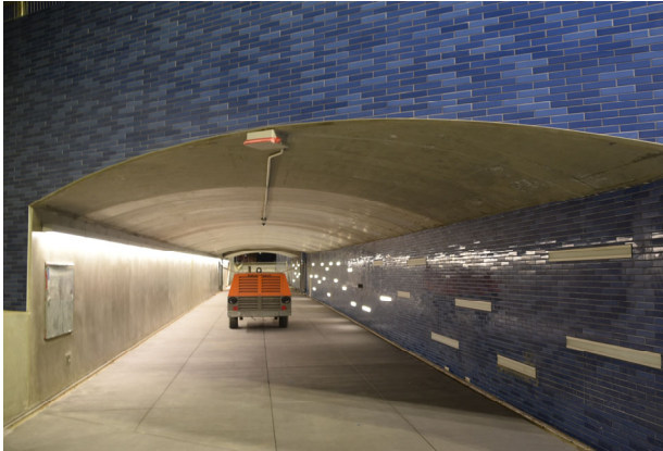
Photo 1 - Ped tunnel looking west
