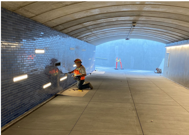
Photo 3 - Ped Underpass looking east
