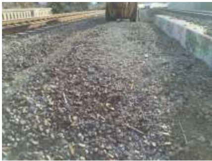
Removed the existing ballast
