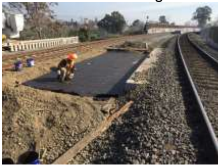
Installed waterproofing material
