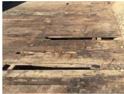
Removed the rotted wooden planks
