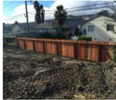
TASI crews removed vegetation. Homeowner replaced fence
