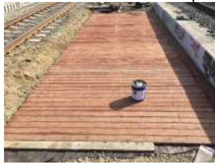
Installed new pressure treated wood planks and reinstalled the existing ballasts
