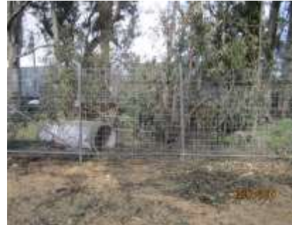
Tree removed and fence repaired
