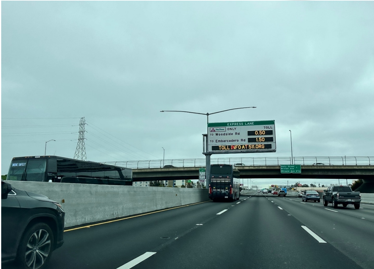
FULLY OPERATIONAL EXPRESS LANES
