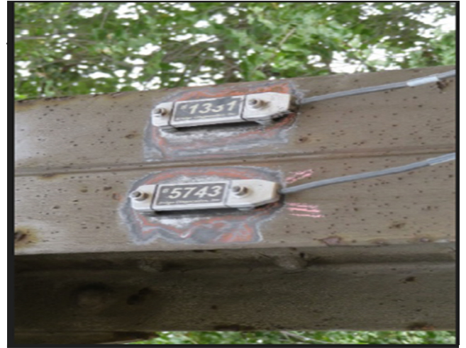
Photo 2 - Strain Gauge on Vertical Members
