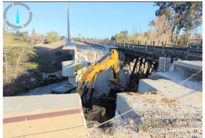
Photo 2 - Preparation for removal of abutment during MT2 partial demolition
