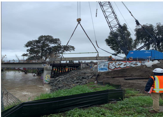
Photo 1 - Existing girder being removed during MT2 partial demolition
