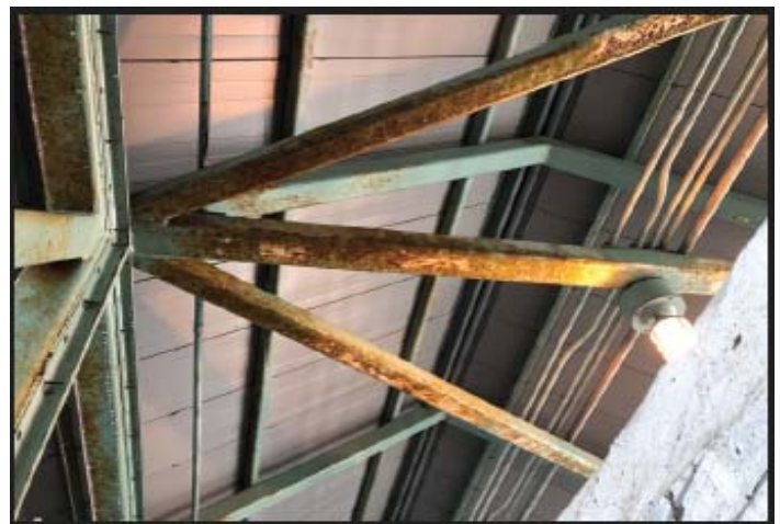
Photo 4 - Post Cleaning - Under Roofside
