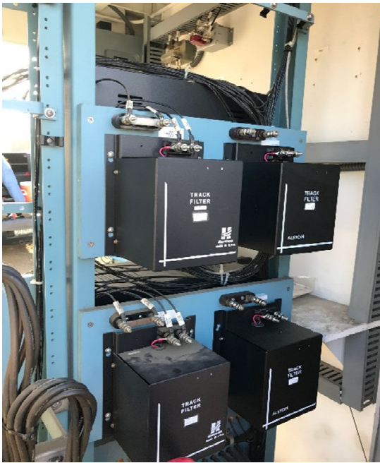
Photo 1 - New advance signal preemption equipment
