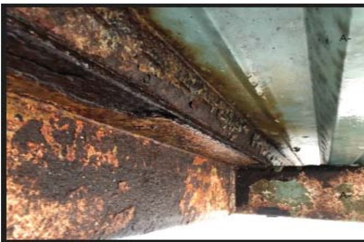
Photo 3 - Post Cleaning - Underside of Pedestrian Bridge
