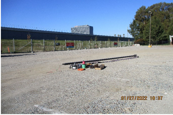
Photo 1 - 25th N Yard Lighting Pole
