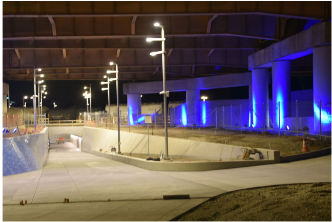
Photo 4 - Poletti Way looking towards East Plaza
