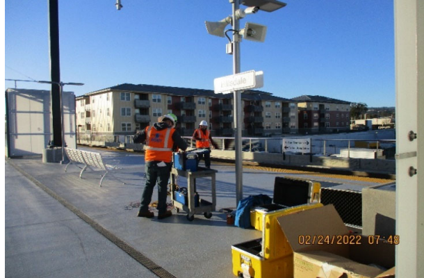
Photo 2 - OCS Grounding Testing.
