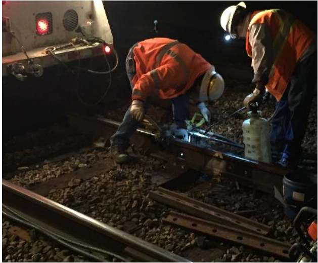
Joint Bars used temporarily to repair the rail defect.
