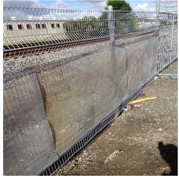
Crews reinforcing existing fence below Curtner Avenue, and the completed fencing
