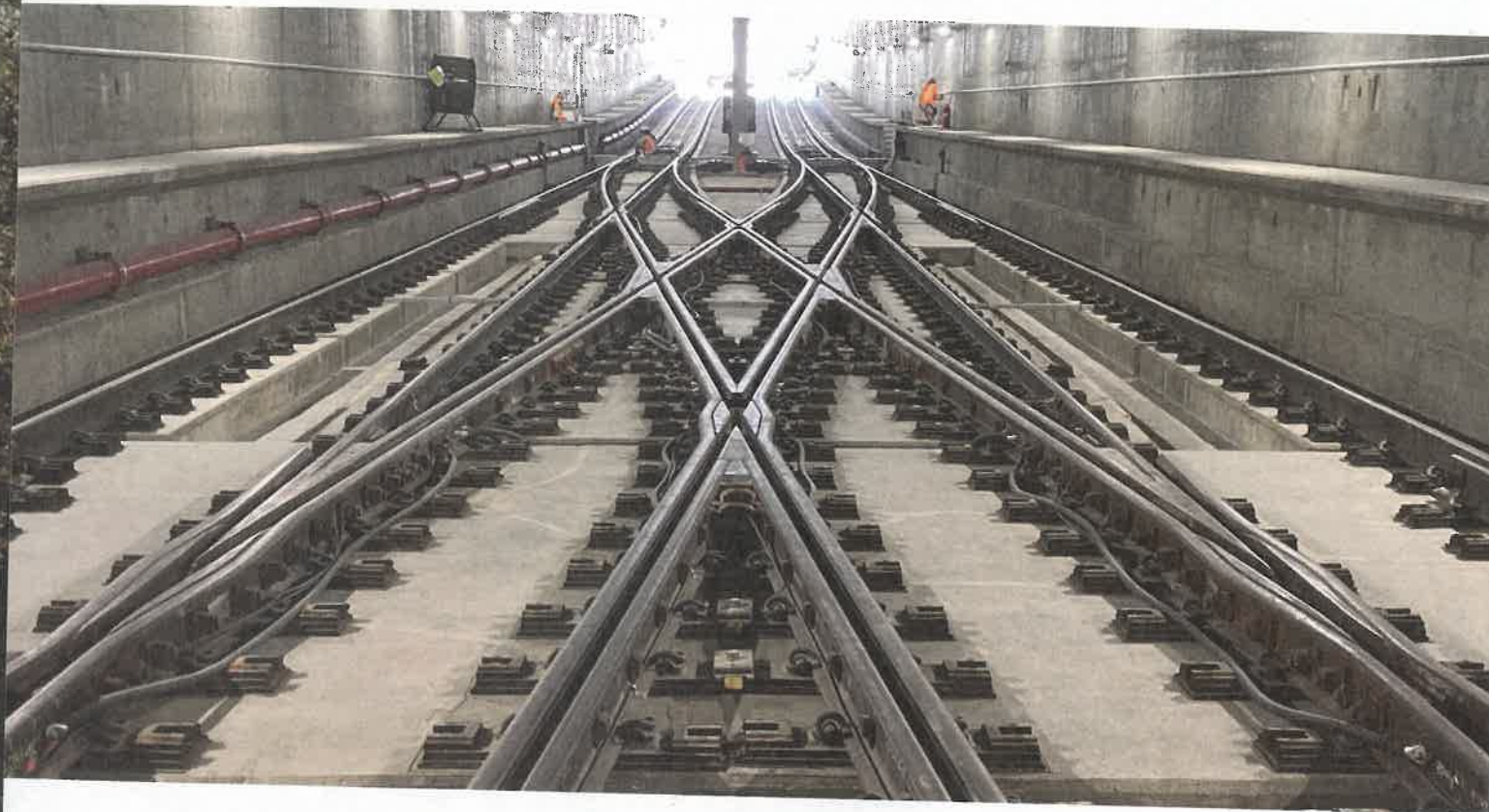
Above shows Voestalpine Railway Systems Nortrak's #10 DXO on Direct Fixation Fasteners for LA Metro.
