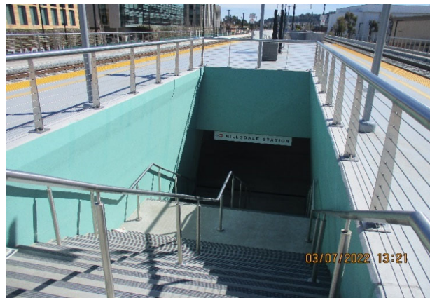
Photo 4 - Stairs Paint Touchup at Hillsdale Station
