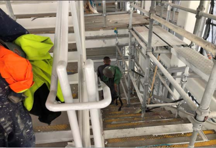
Photo 3 - West Tower Paint Layer
