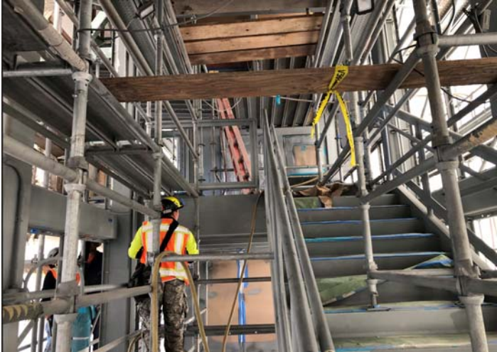
Photo 4 - East Tower Paint Preparation
