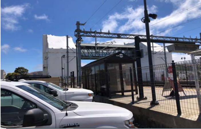
Photo 2 - East Side Containment System
