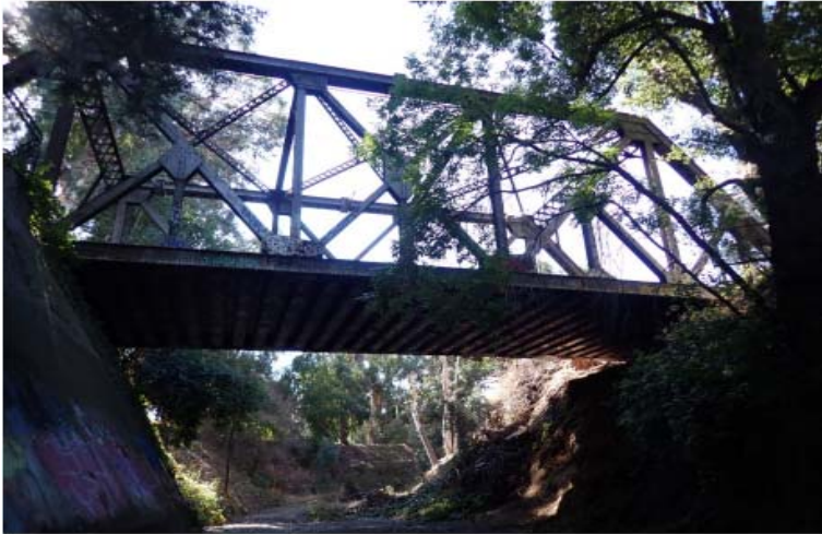
Photo 1 - Bridge West View
