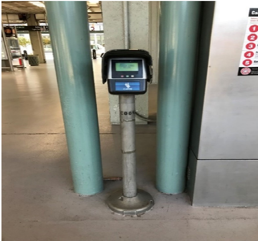
Photo 1 - Old Clipper CID removed via Change Order
