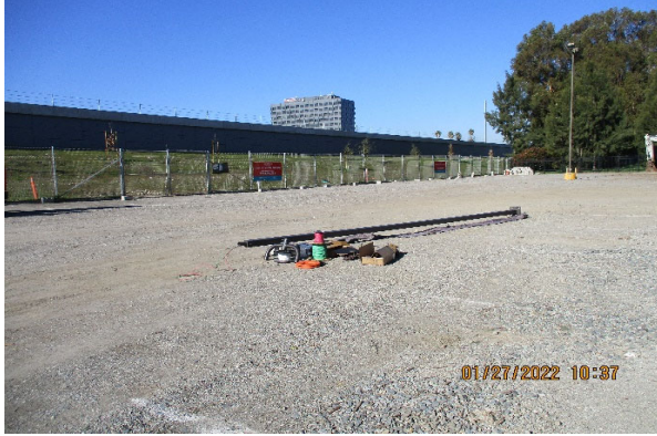
Photo 1 - 25th N Yard Lighting Pole
