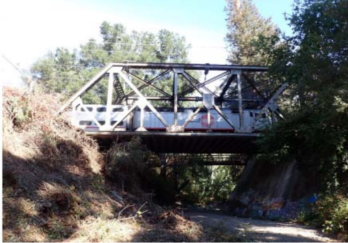
Photo 2 - Bridge East View
