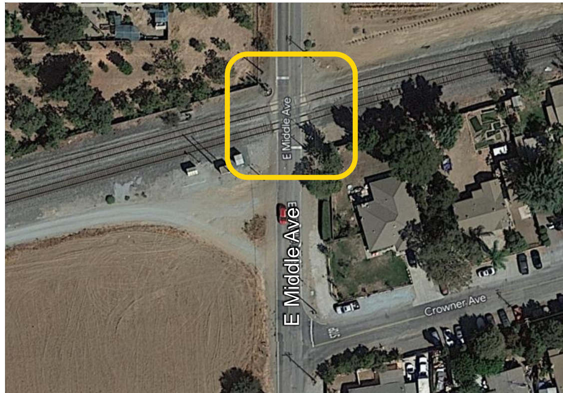
E Middle Ave Crossing, Morgan Hill
