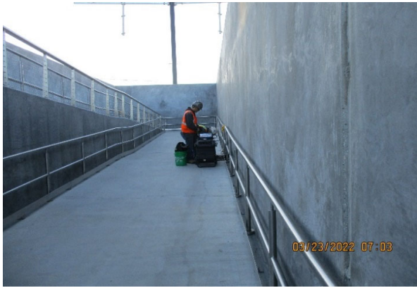
Photo 3 - South Ramp fixing plate kickers
