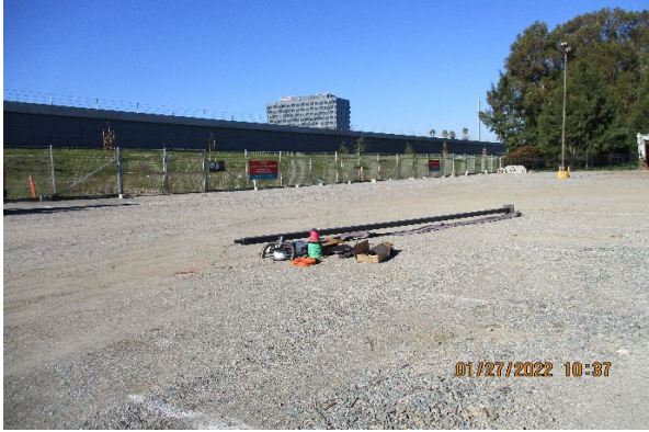
Photo 1 - 25th N Yard Lighting Pole
