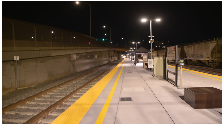
Photo 4 - New platform looking north MT-2
