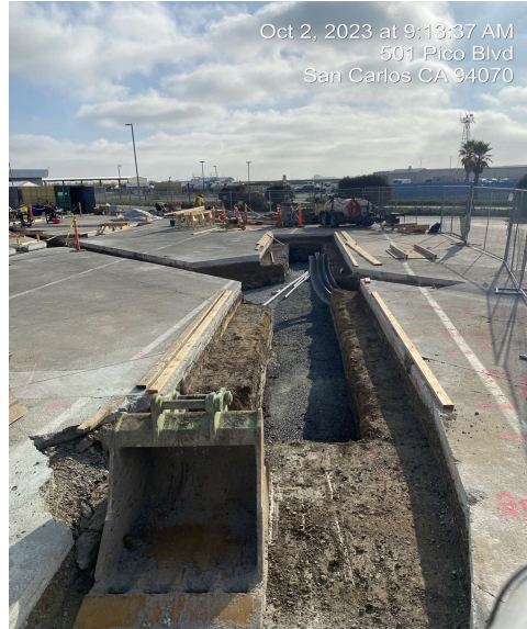
Within South Base's "Deadline" Area, excavation for the new Chargers' foundations, dispenser's foundations, and trenches were completed.
