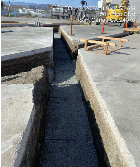
Within South Base's "Deadline" Area, excavation for the new Chargers' foundations, dispenser's foundations, and trenches were completed.
