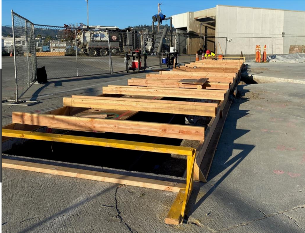
Construction of Charger Pads.
