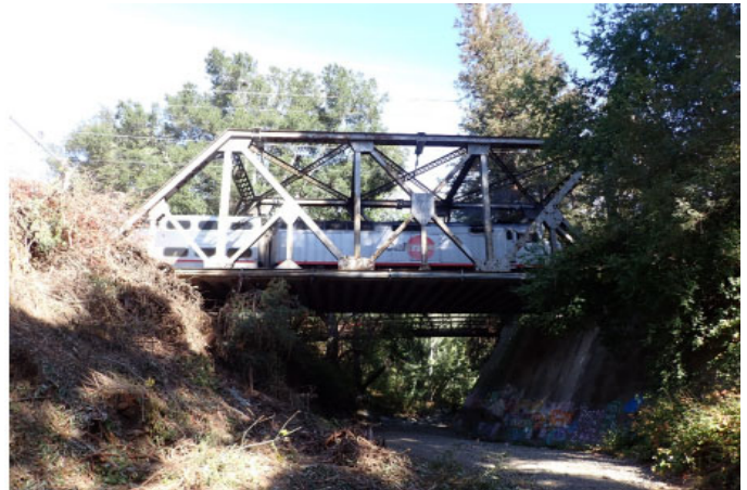
Photo 2 - Bridge East View
