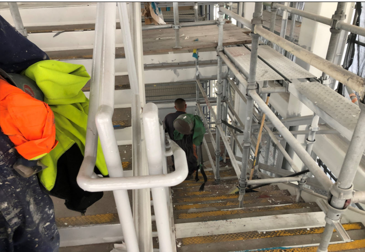
Photo 3 - West Tower Paint Layer
