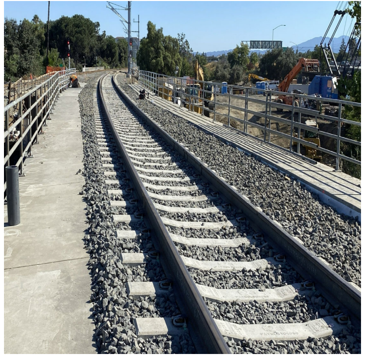
Photo 2 - New track on erected MT2 bridge
