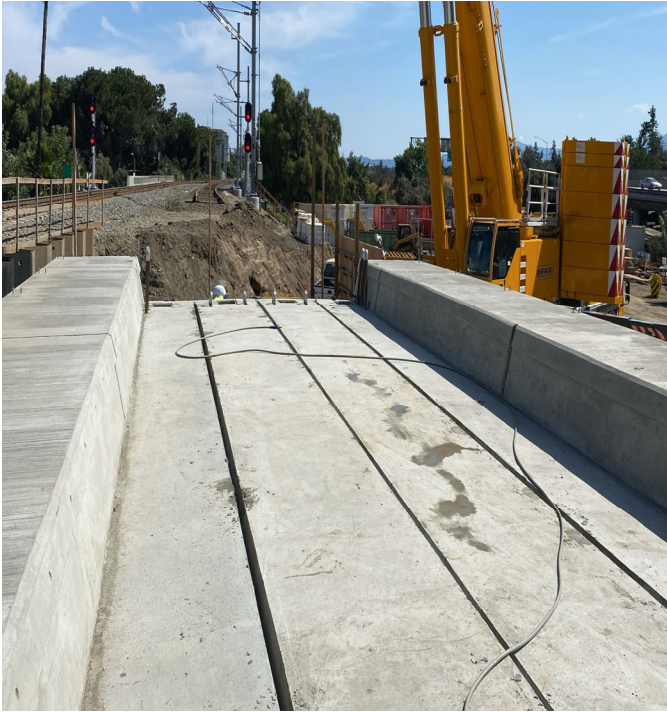
Photo 1 - Partially erected MT2 bridge
