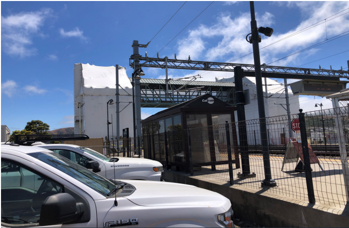
Photo 2 - East Side Containment System
