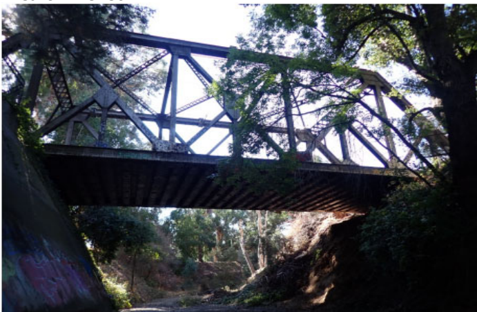
Photo 1 - Bridge West View
