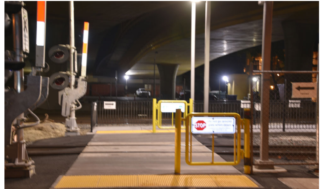
Photo 2 - Ped grade crossing
