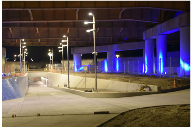
Photo 4 - Poletti Way looking towards East Plaza
