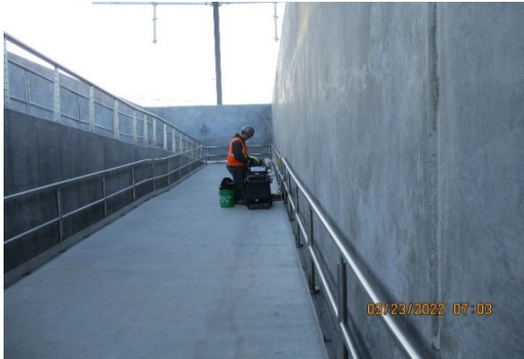
Photo 3 - South Ramp fixing plate kickers
