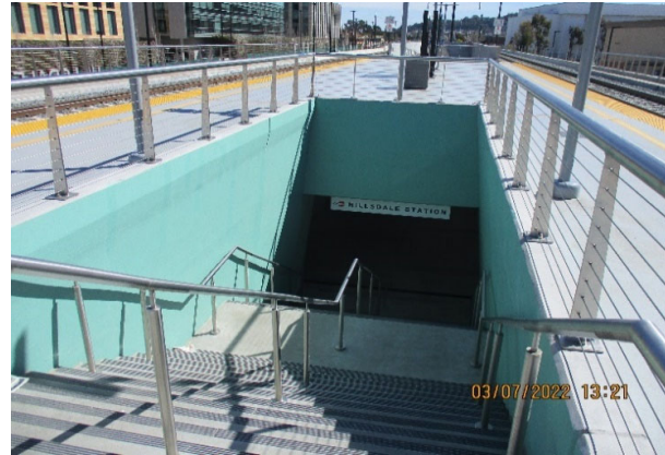
Photo 4 - Stairs Paint Touchup at Hillside Station
