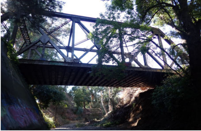
Photo 1 - Bridge West View
