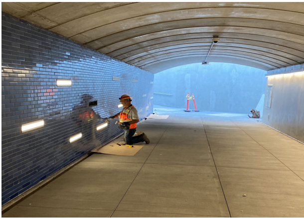
Photo 3 - Ped Underpass looking east
