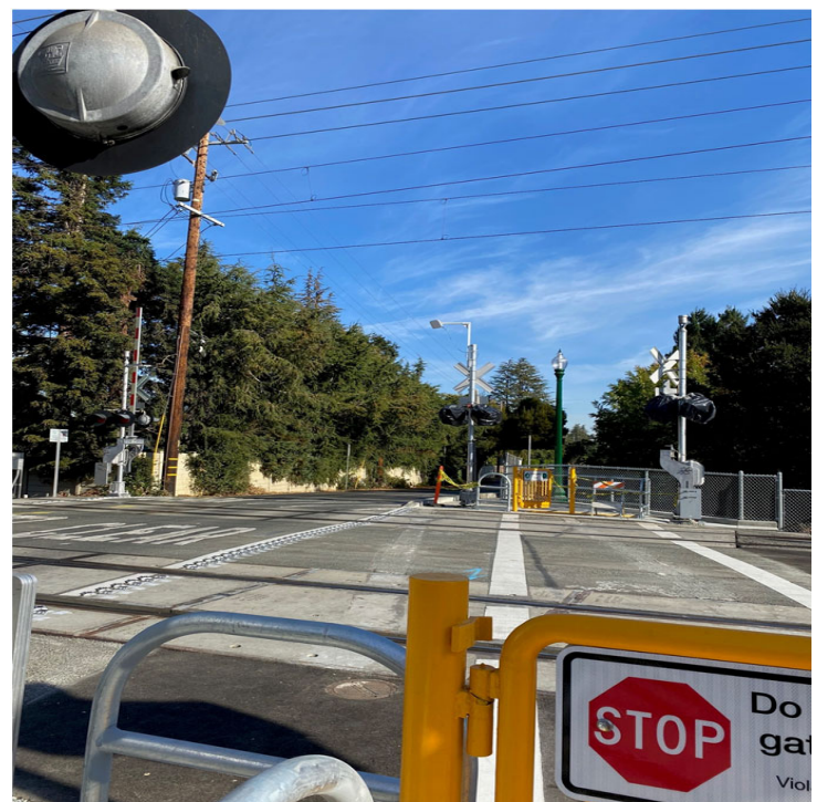
Newly installed exit gates
