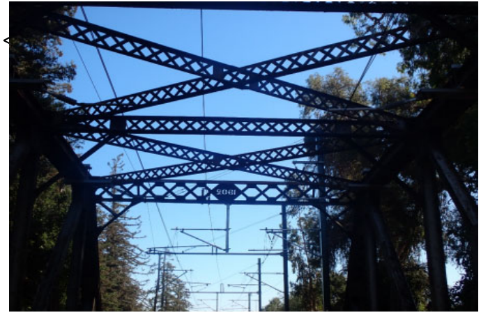
Photo 4 - OCS Installed
