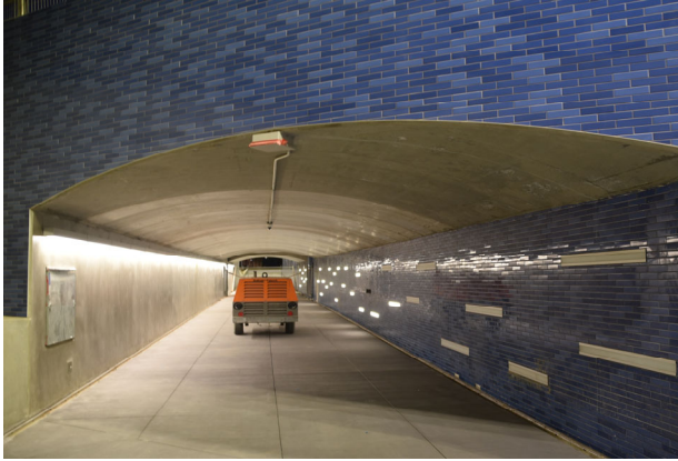
Photo 1 - Ped tunnel looking west
