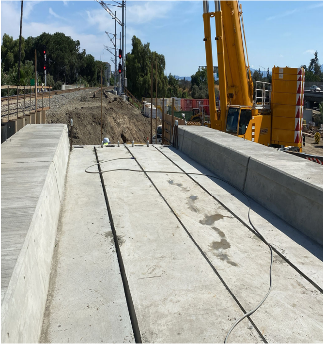
Photo 1 - Partially erected MT2 bridge
