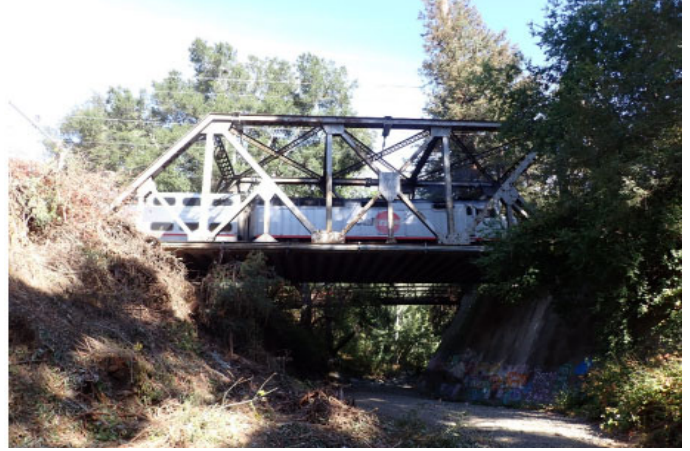
Photo 2 - Bridge East View
