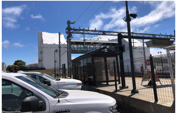
Photo 2 - East Side Containment System
