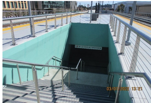
Photo 4 - Stairs Paint Touchup at Hillsdale Station
