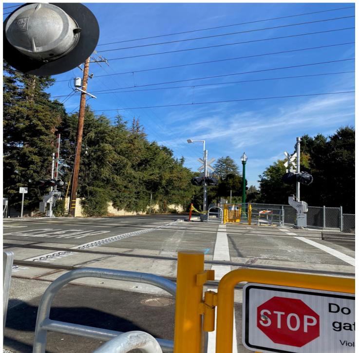
Newly installed exit gates
