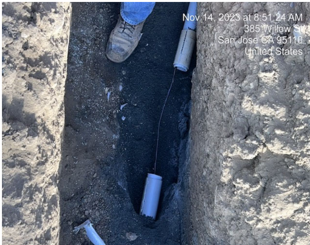
Photo 1 - Trenching and Conduit for the electrical power cable to the Broadband Radio.
