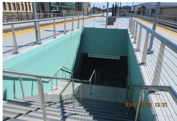
Photo 4 - Stairs Paint Touchup at Hillsdale Station
