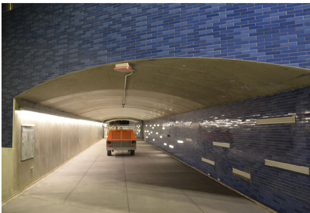
Photo 1 - Ped tunnel looking west
