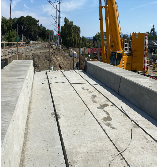
Photo 1 - Partially erected MT2 bridge
