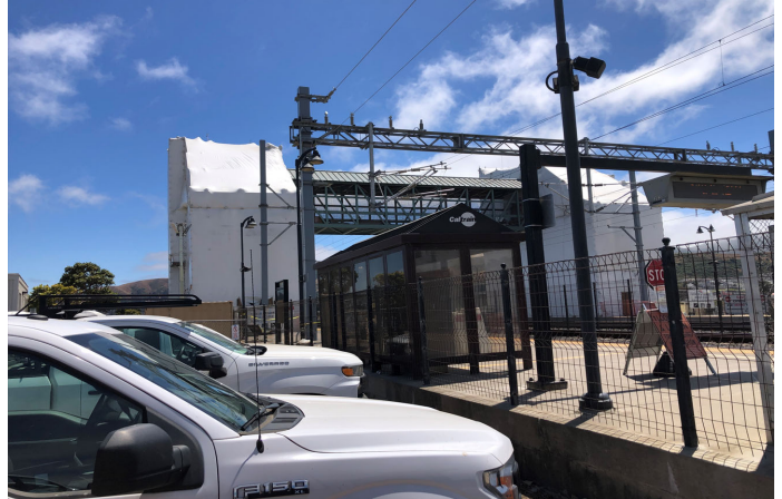
Photo 2 - East Side Containment System
