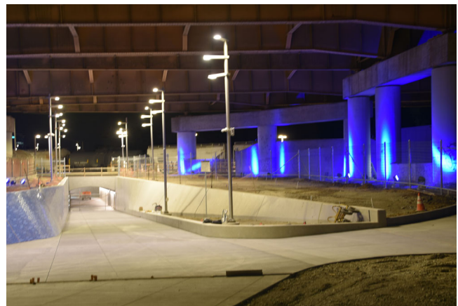
Photo 4 - Poletti Way looking towards East Plaza
