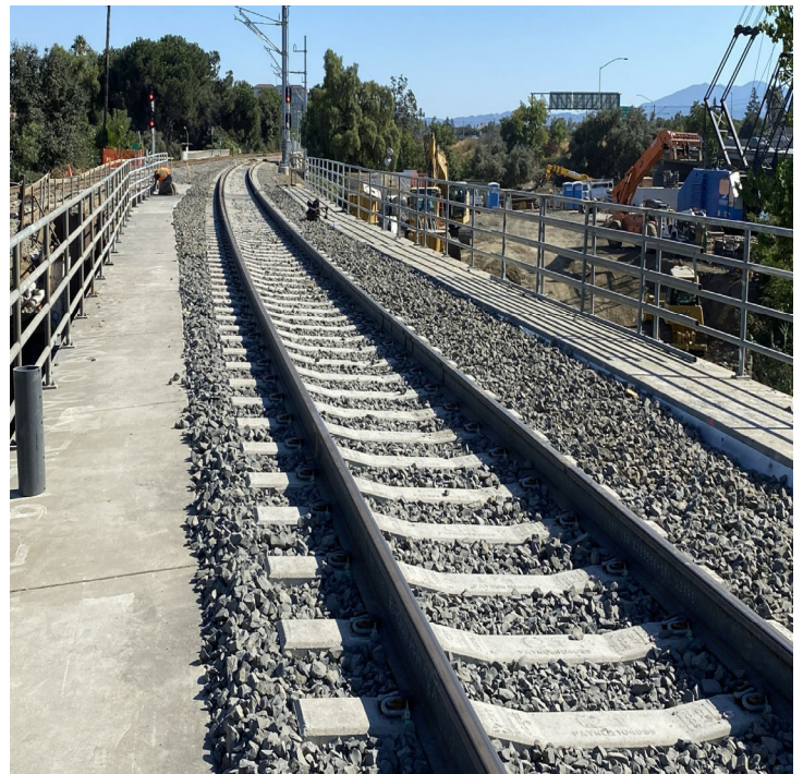
Photo 2 - New track on erected MT2 bridge
