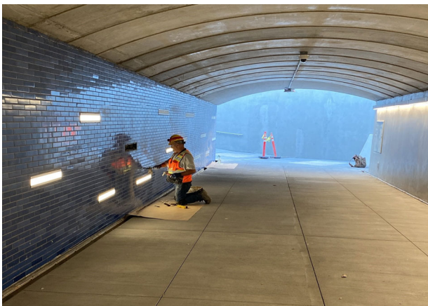
Photo 3 - Ped Underpass looking east
