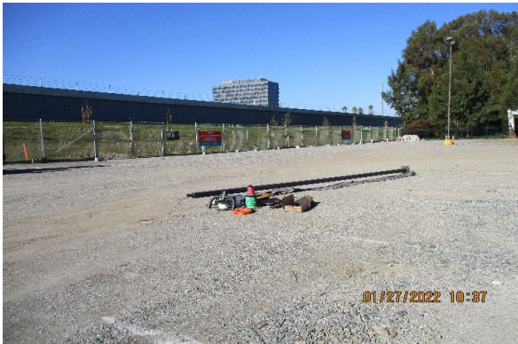
Photo 1 - 25th N Yard Lighting Pole
