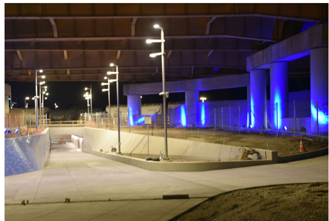
Photo 4 - Poletti Way looking towards East Plaza
