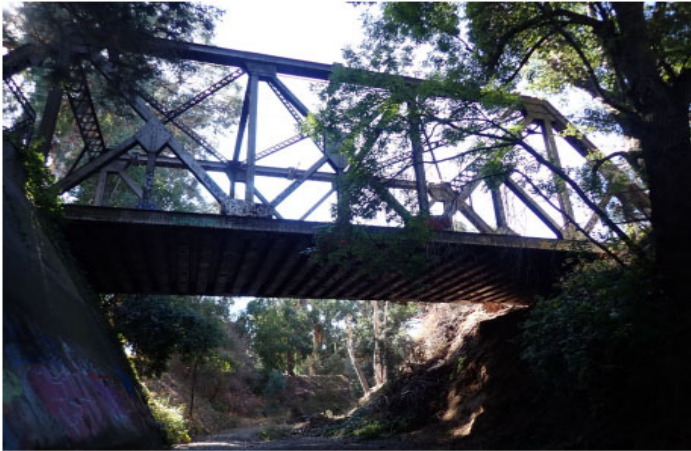
Photo 1 - Bridge West View
