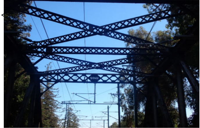
Photo 4 - OCS Installed
