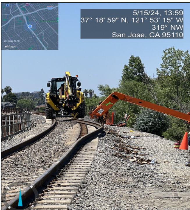
Photo 1 - Rail removal MT1
