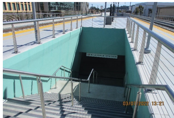
Photo 4 - Stairs Paint Touchup at Hillsdale Station
