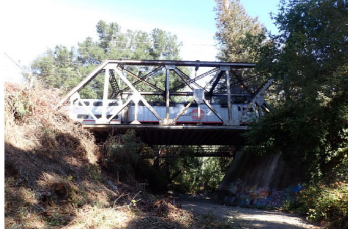
Photo 2 - Bridge East View
