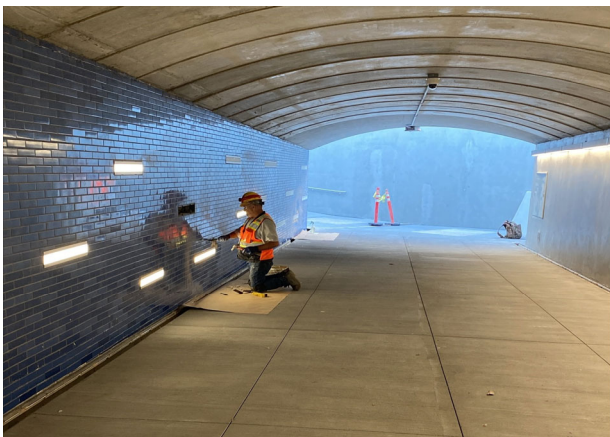
Photo 3 - Ped Underpass looking east
