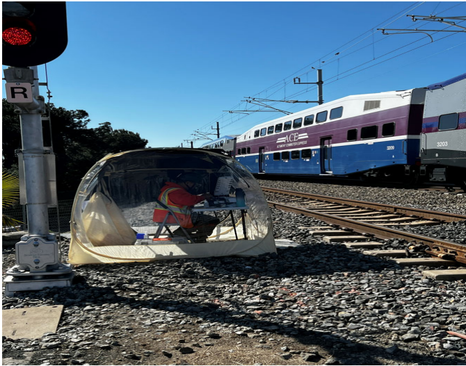
Photo 3 - Fiber Optic cable testing
