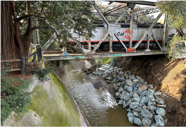
Temporary stabilization measures currently in place
