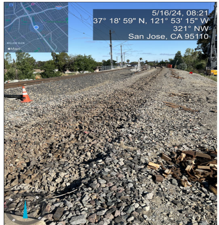
Photo 2 - Rail removed from MT1
