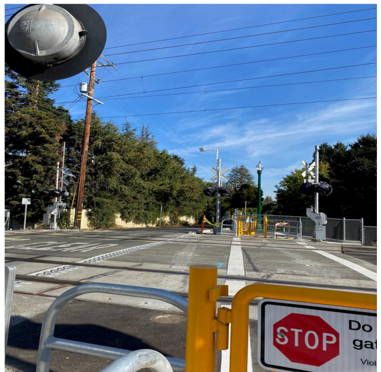
Newly installed exit gates
