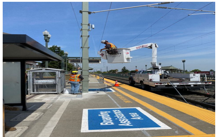
Photo 2 - Installing antenna on OCS pole at San Carlos station
