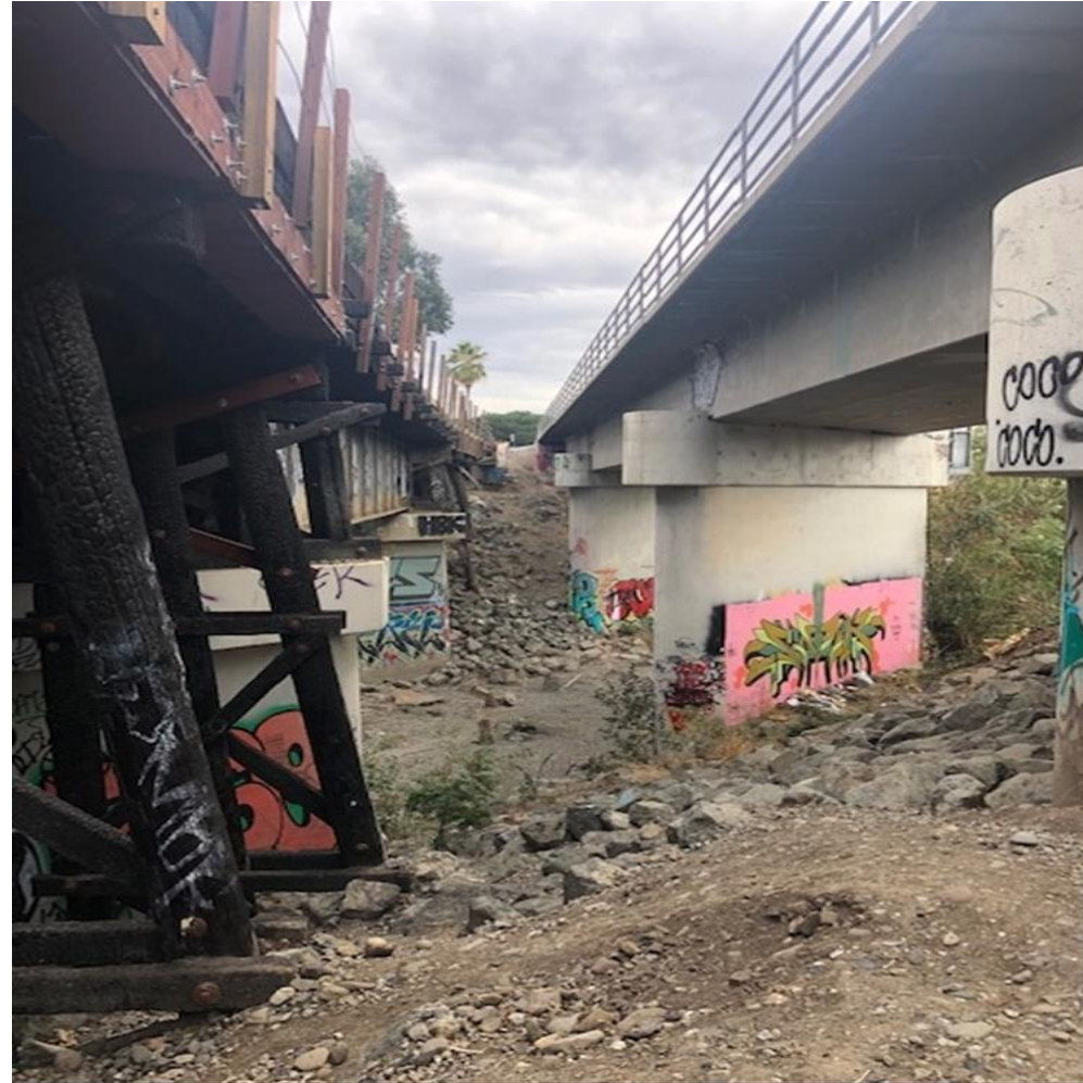
Northbound MT-1 (1935); Southbound MT-2 (1990)
