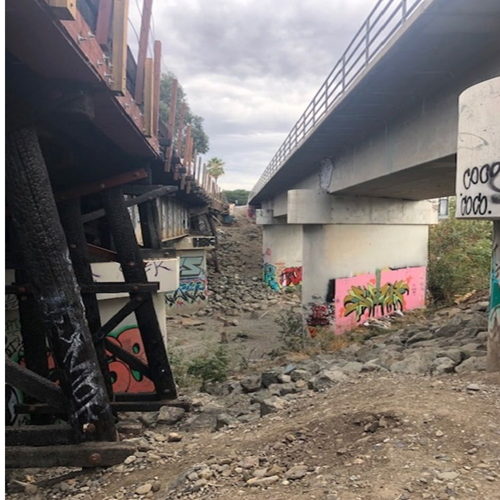
Northbound MT-1 (1935); Southbound MT-2 (1990)
