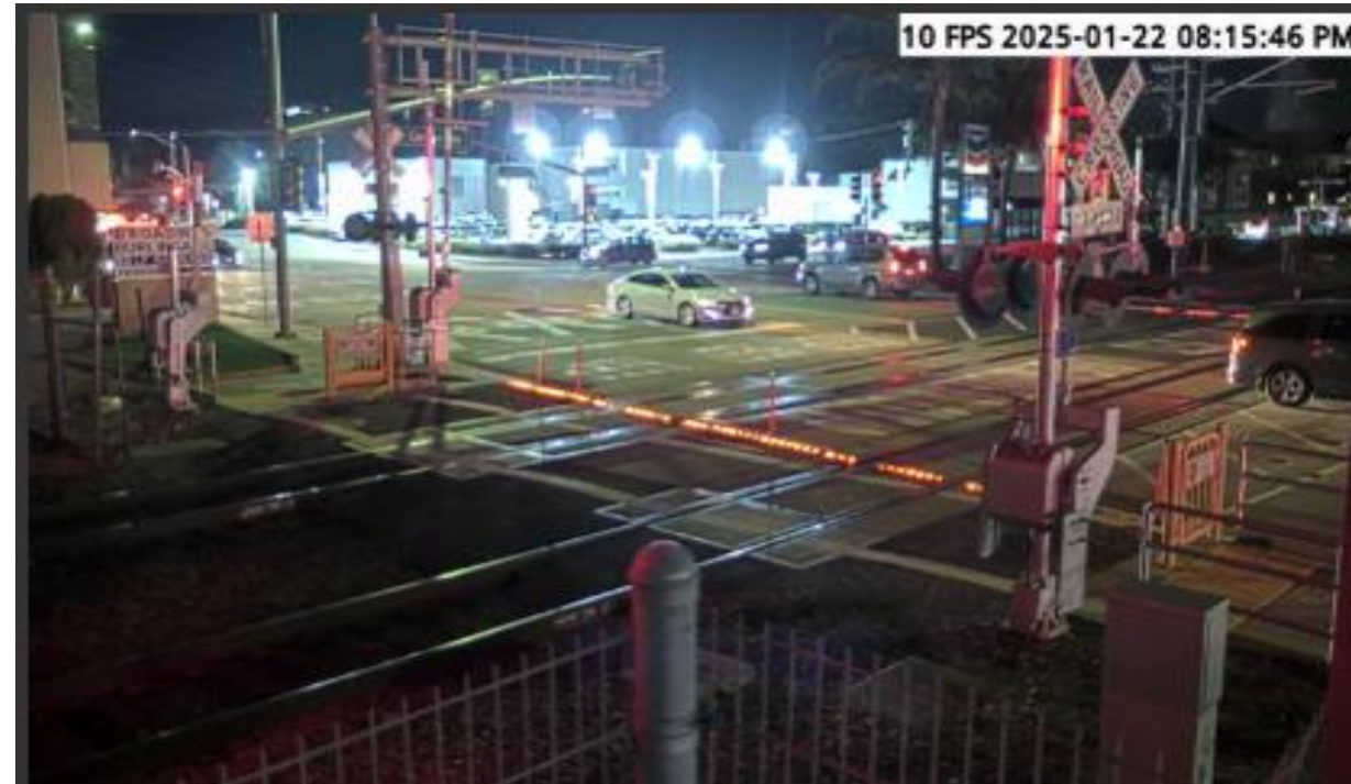
Broadway Crossing with Solar Markers and Delineators
