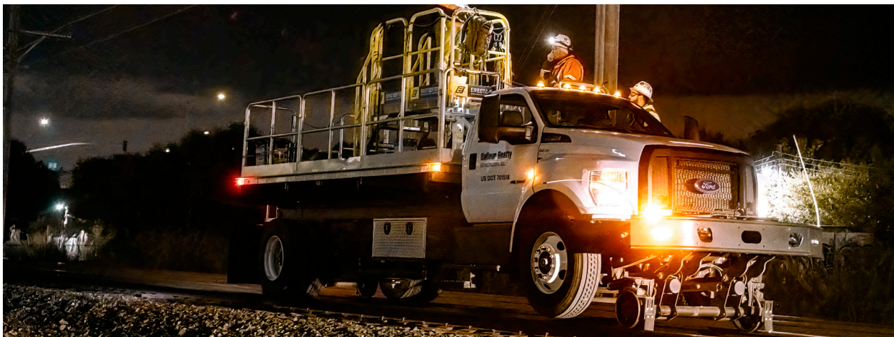
Balfour Beatty Night Wire Work
