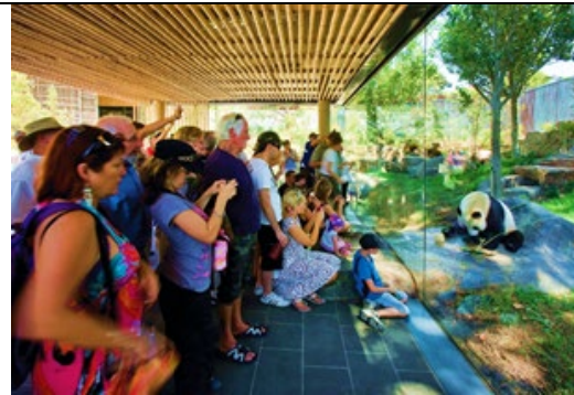
Adelaide Zoo Bamboo Forest: Visitors flow through a sequence of rooms, both indoor and outdoor, for a series of experiences---duck water glades to circular amphitheater spaces. The 55,400 square feet facility has a separate conservation center---research, breeding, and education. https://architectureau.com/articles/giant-panda-bamboo-forest-adelaide-zoo/
