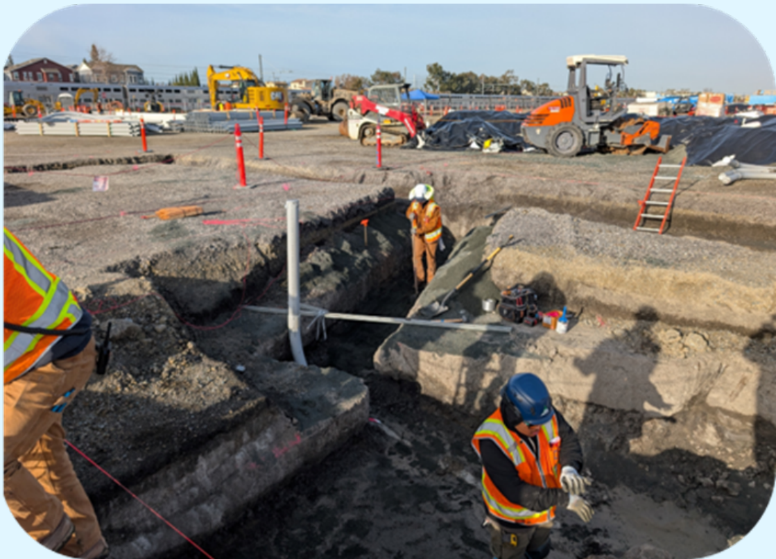
Installing lateral utility connections
