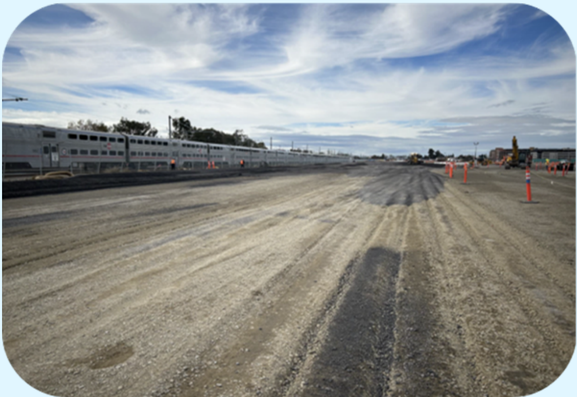
Grading complete for top of launch structure
