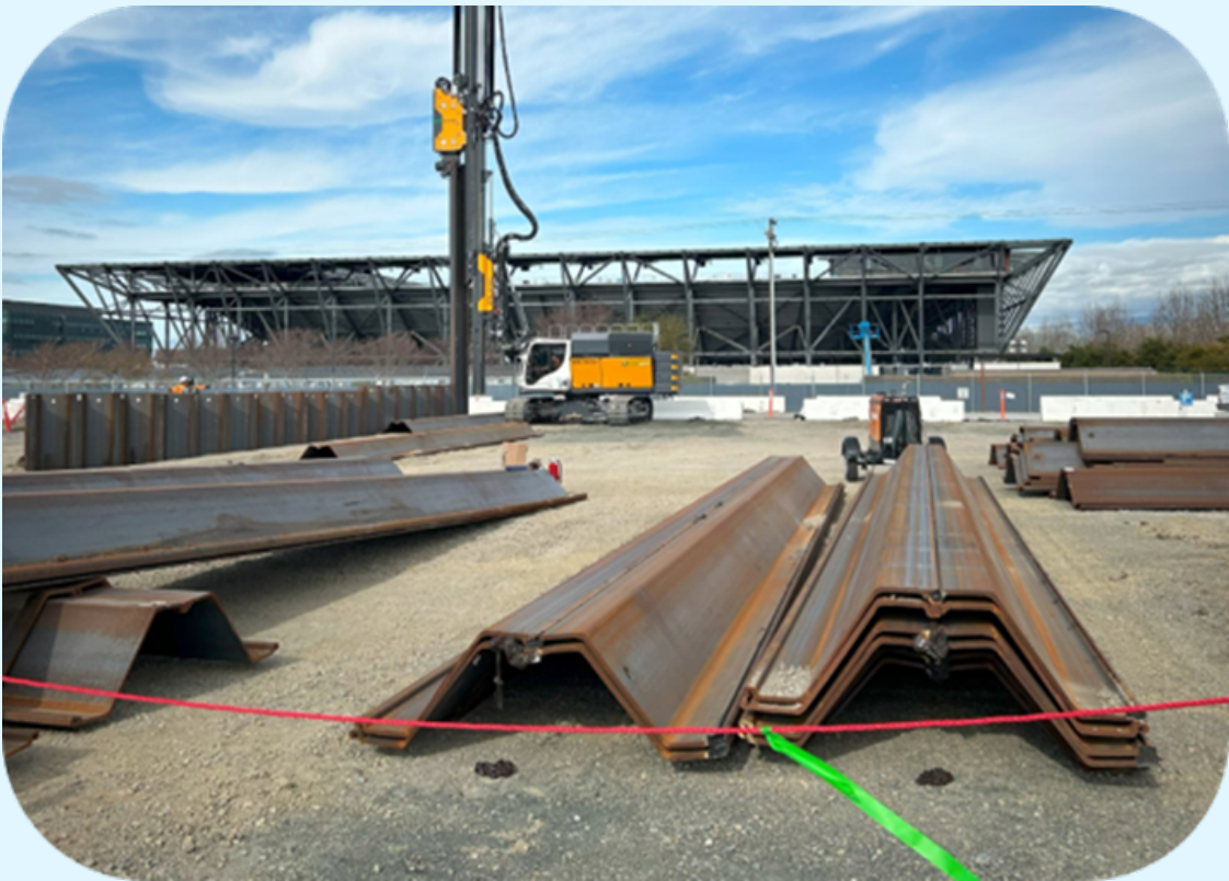
Prepared and installed sheet piling for detention basin
