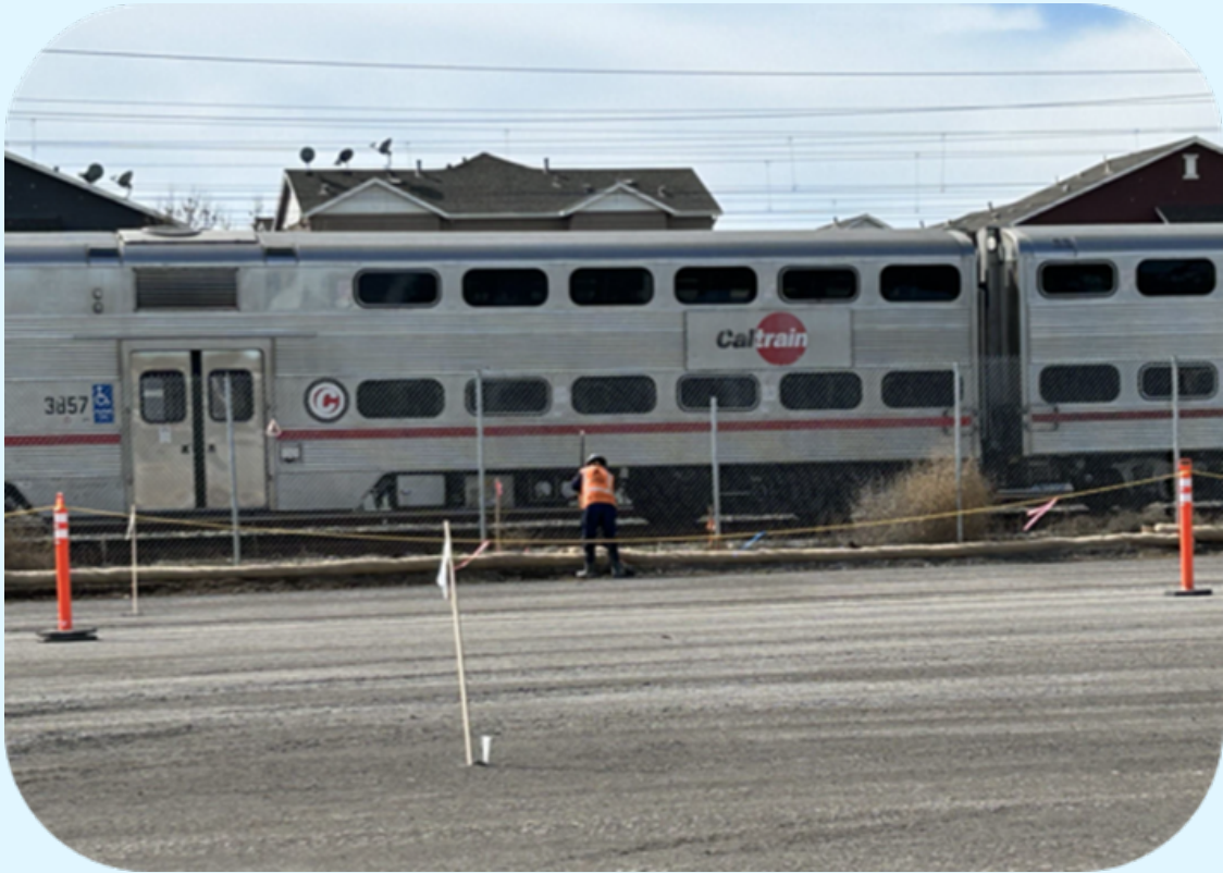
Survey checks for instrumentation and monitoring
