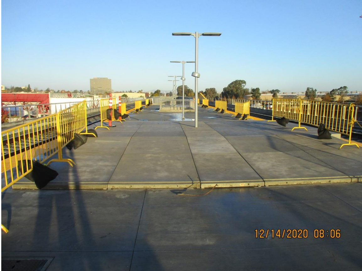
Mini-high at Center Island Platform
