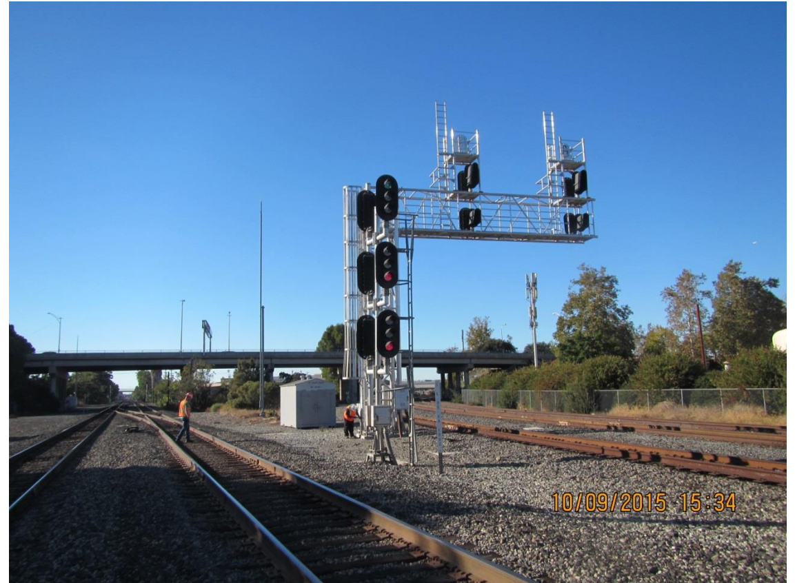
Signal Cantilever
