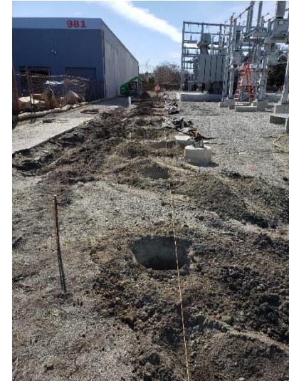
Excavating for site fence foundations at TPS-2.
