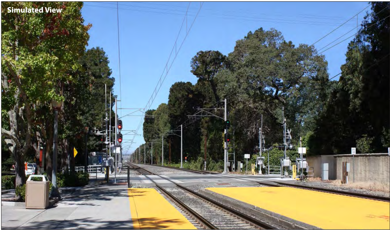
Looking northwest down the rail corridor with the OCS system and tree trimming, as seen from the Atherton Caltrain Station platform near Fair Oaks Lane.
