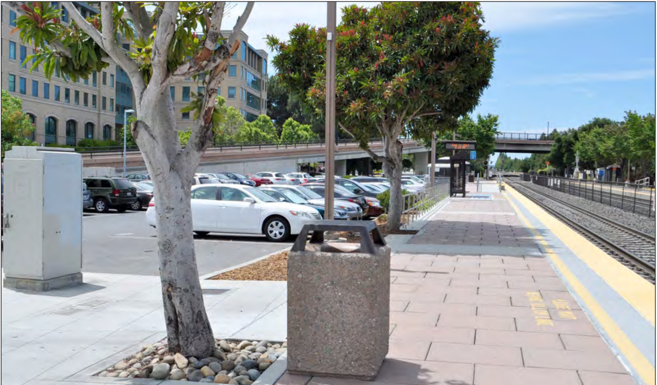
Photo 16, PS6 Option 2. Looking northwest from the Sunnyvale Caltrain station plaza toward the rail corridor and PS6 Option 2.
