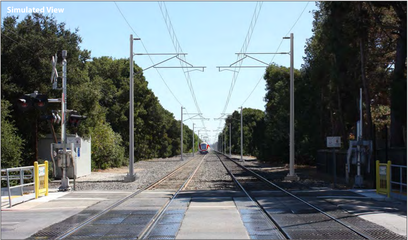
Looking southeast down the rail corridor with the OCS system and tree trimming, as seen from Churchill Avenue.
