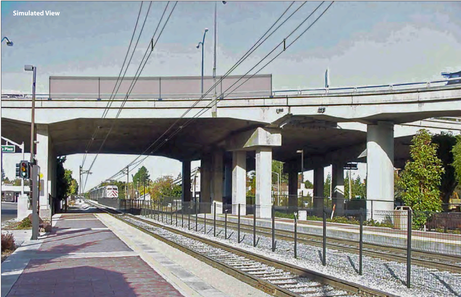
Looking northwest down the rail corridor with the OCS system and overbridge protection barrier, as seen from the San Antonio Caltrain Station platform.
