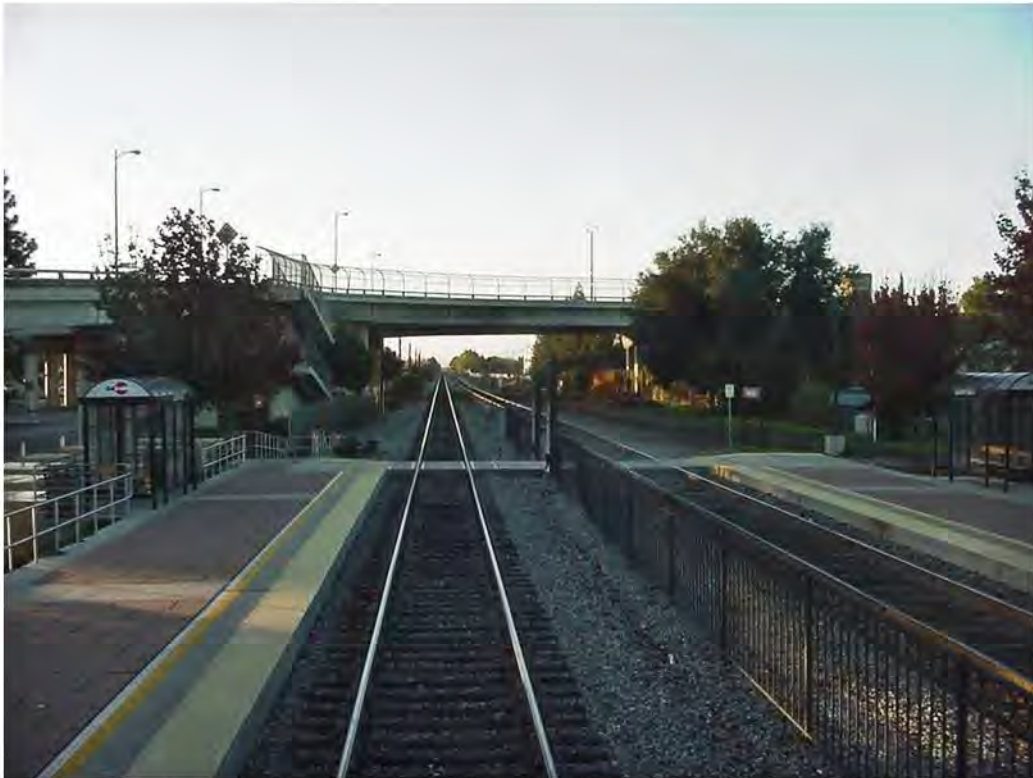
Existing Caltrain Pedestrian Walkway with Overbridge Protection Barrier
