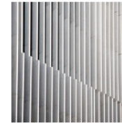
Vertical Aluminum Louvers on West Facades
