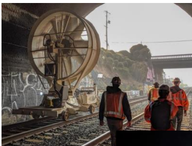
Fan used to maintain airflow during notching
