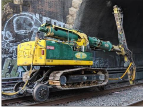
On-Track Drill (for Rock Bolts and Grout Holes)
