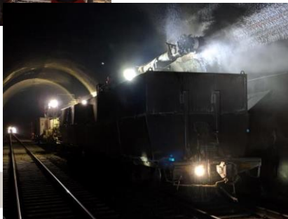
Roadheader Notching Operation
