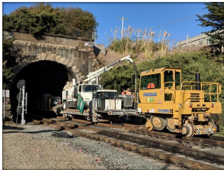
South Portal MT1 Potholing for OCS Termination Structure Piles
