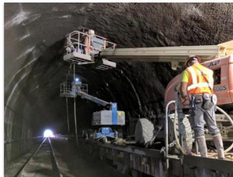
Grouting Operation
