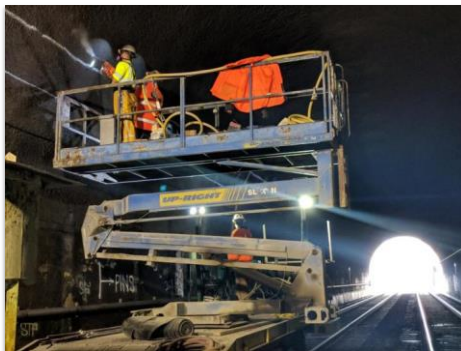
Dry Fix Pin Installation
