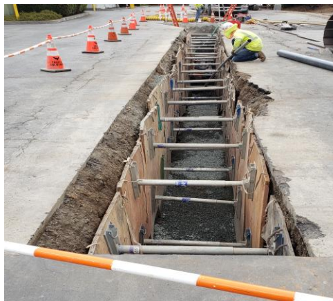
Drainrock Installation for the Circuit #2 Ductbank in the HealthPeak Parking Lot
