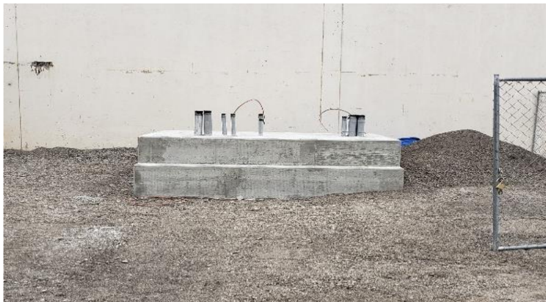
PS-3 – Poured auxiliary pad.
