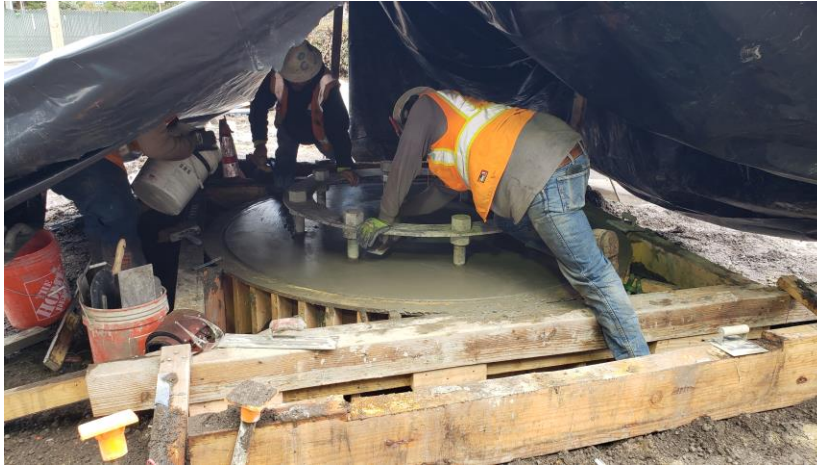
TRC Installing TSP Foundation in HealthPeak Parking Lot
