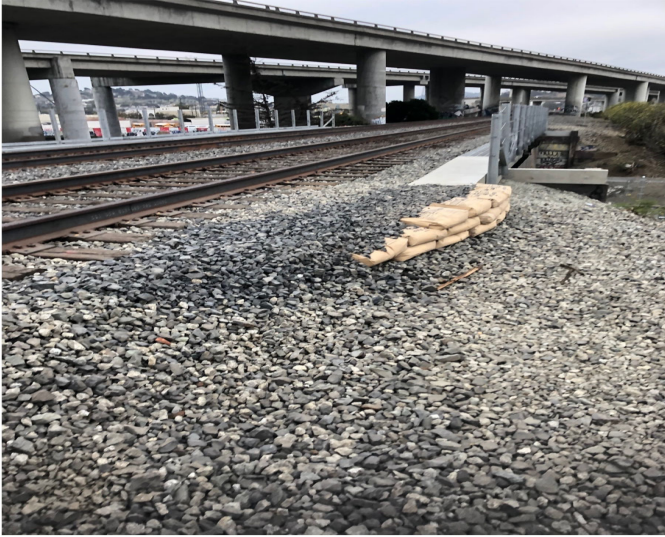
Photo 1 - Marin Street New Walkways
