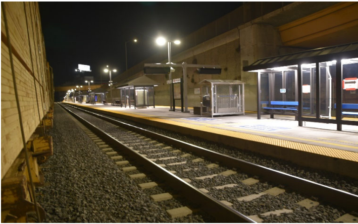
Photo 1 - New platform looking south
