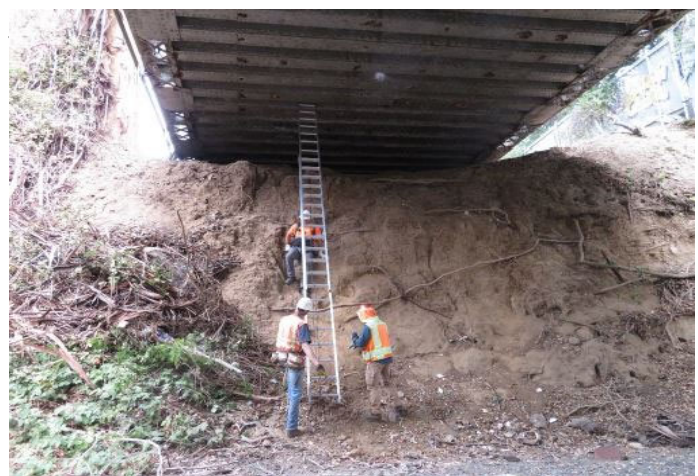
Photo 4 - Inspection crew via north side abutment
