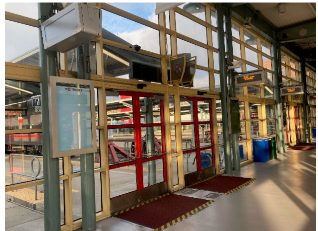
Photo 4 - Doors 5, 6, 7 and 8 APC
