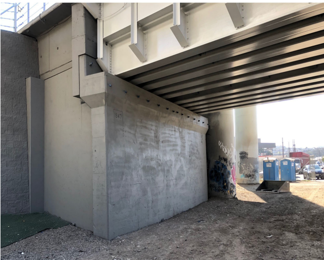
Photo 3 - Napoleon South Abutment
