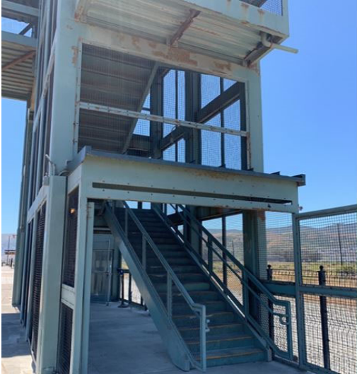
Photo 3 - Stair Case (west side)
