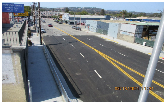
Photo 4 - 25th Ave. Opening
