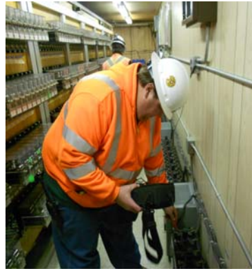
Performing end of work ground verification test
