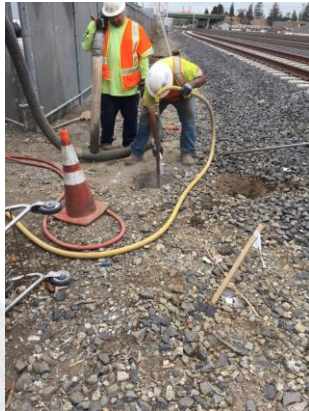
Potholing – to identify utilities
