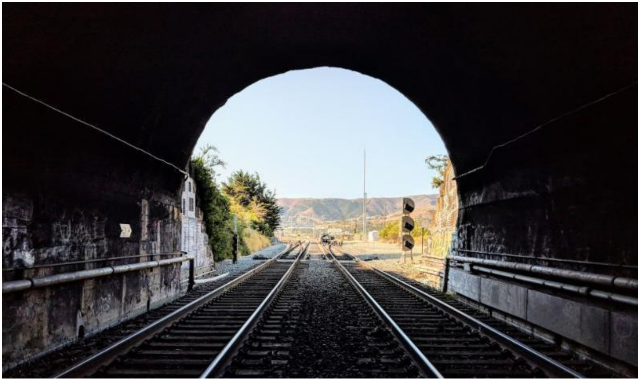
Inside one of the SF Tunnels looking South
