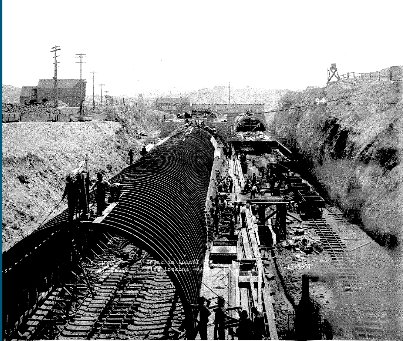
Bayshore Tunnels under construction, 1907
