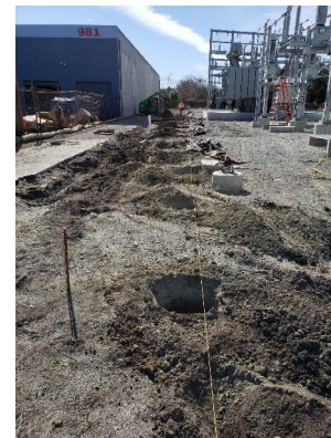
Excavating for site fence foundations at TPS-2.
