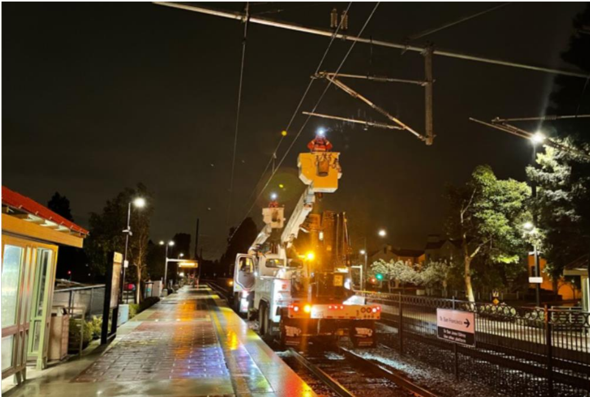
Installation of overhead wire at a Caltrain Station
